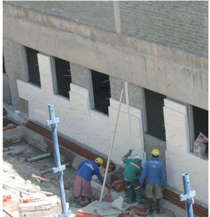
Double layer wall insulation, Maun Hospital
