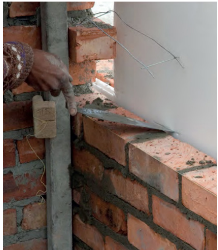
Double layer wall insulation, Maun Hospital
