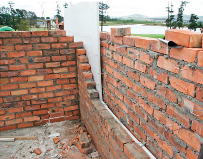
Double layer wall insulation, Maun Hospital
