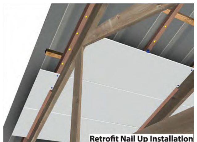
Retrofit nail up installation
