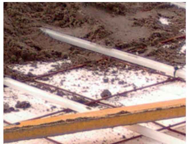
Above slab, below screed insulation
