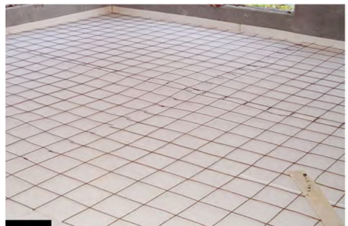
^ IsoBoard installation over slab under screed
